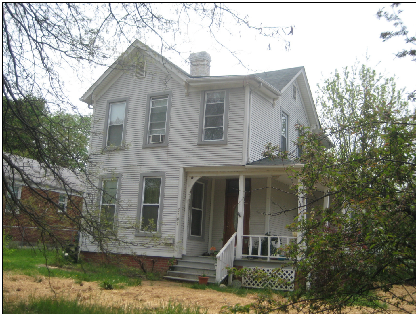
Photo: Hall House, Berwyn Heights, façade (north elevation), view looking southeast. (April 2008)
