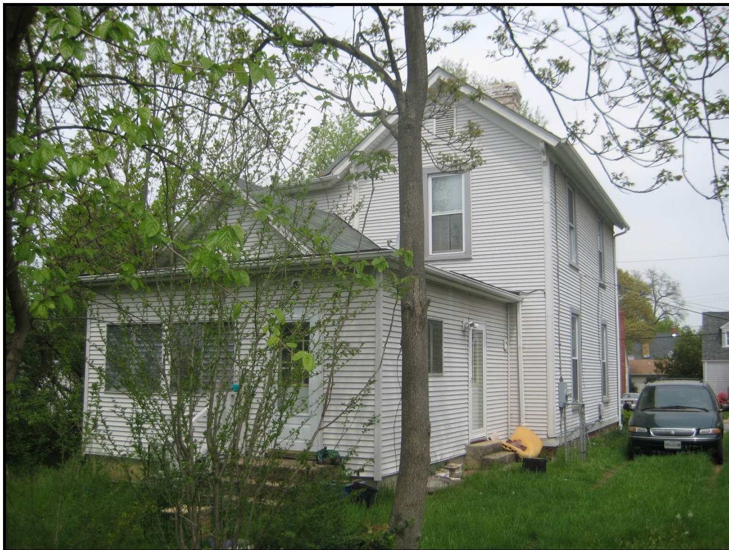
Photo: Hall House, Berwyn Heights, rear (south) elevation, view looking northwest. (April 2008)
